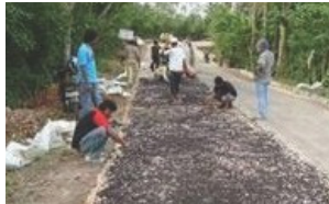
(3) Asbuton spread out
