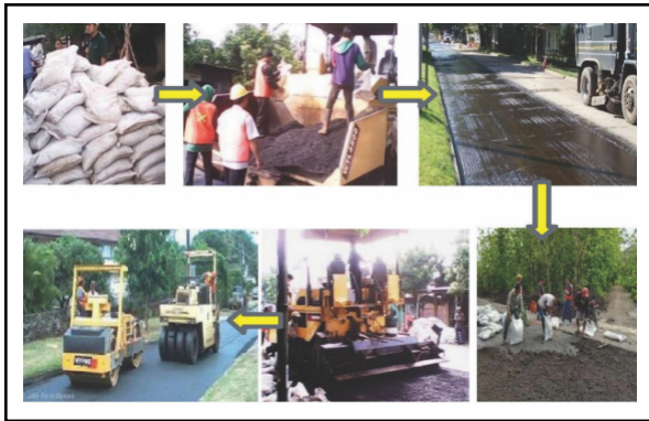
Gambar 3.5 Perkerasan jalan Cold Paving Hot Mix Asbuton (CPHMA).
